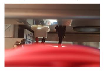
Locate and connect the matching plugs in the right hand side of the HS module - behind the panel with contactors. Black 3-pole plug L1 / L2 / L3 and white 9 pole plug 4L1 / 4L2 / 4 L3 / 3L1 / 3L2B.
